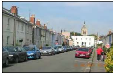
Figure 18 View down Francis Street stopped by buildings on Bath Road (note steeple of St Phillip & St James Church in background)
