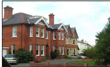
Figure 3 Grand historic houses along Leckhampton Road
