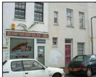
Figure 22 Car repair garage on St. Luke's Road
