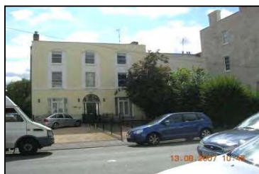
Figure 35 Rendered building on Bath Road
