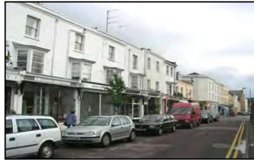
Figure 29 Shops occupying ground floor of 27 to 34 Suffolk Parade
