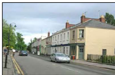
Figure 11 Buildings front directly onto back edge of footpath along Suffolk Road
