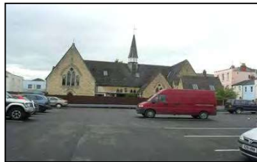
Figure 32 Former St James's School building
