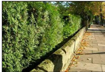
Figure 21 Historic stone plinth on Queen's Road. Note where the railings used to be.
