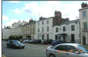
Figure 21 Businesses in the character area
