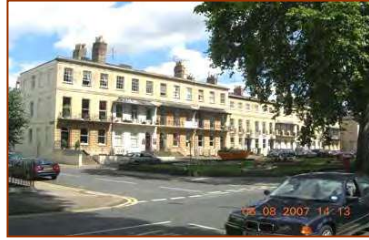
Figure 25 Listed terraced houses on Priory Parade, London Road
