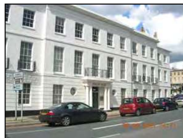
Figure 7 Stirling House, High Street/College Road
