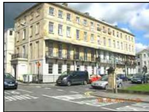
Figure 37 Ashlar faced terrace, London Road
