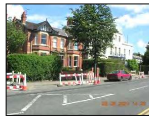
Figure 39 Brick faced villa, London Road
