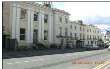
Figure 12 Railings on London Road
