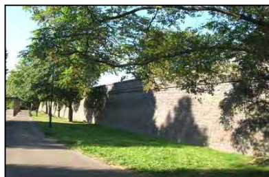
Figure 11 High brick wall of railway embankment
