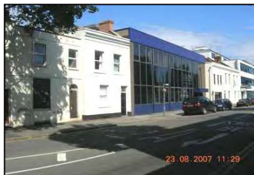
Figure 33 CPS building on Ambrose Street
