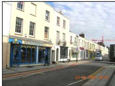
Figure 29 Listed terraced houses on Henrietta Street
