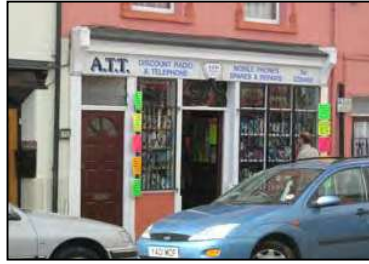
Figure 28 Detailing on historic shop front on Lower High Street
