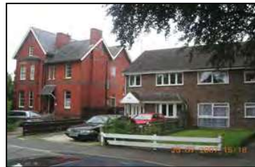
Figure 32 Modern building (to right) on All Saints Villas
