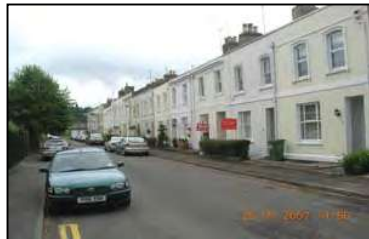
Figure 22 All Saints Terrace – a residential street
