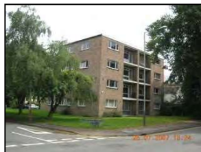
Figure 47 Poor quality modern block on All Saints Road
