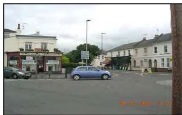
Figure 23 Shops on Hewlett Road
