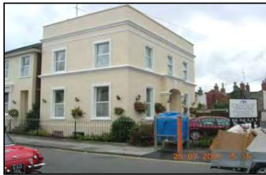
Figure 40 Building finished in stucco in All Saints' Road
