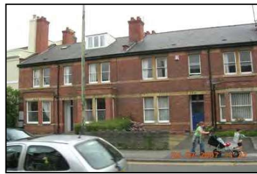
Figure 41 Terraces with facing brick in Hewlett Road
