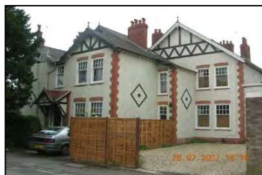
Figure 16 Poor wooden fencing evident in All Saints Villas Road
