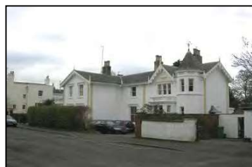
Figure 21 Hard standing evident outside house on Ashford Road
