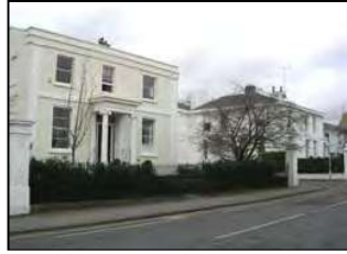
Figure 35 Neo-Classical style of architecture on villas in Park Place
