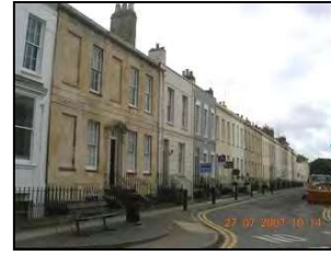
Figure 34 Albert Place terraces
