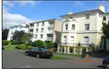
Figure 17 Modern and historic buildings on East Approach Drive follow similar building line
