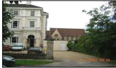
Figure 25 View of All Saints Church from Pittville Circus Road
