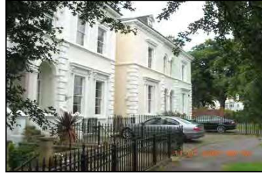
Figure 20 Hard-standing on Pittville Crescent
