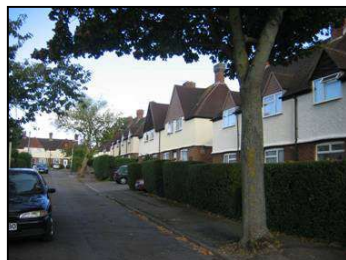
Figure 31 Timber cladding under gables of houses on Shelley Avenue
