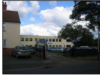
Figure 26 Spirax Sarco site on Tennyson Road
