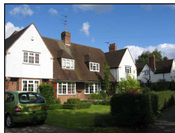
Figure 42 Shallow dormer windows on roof slopes of houses in Kingsley Gardens
