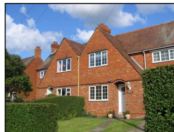
Figure 32 Low rooflines of houses on Tennyson Road
