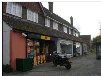
Figure 2 The shops on Tennyson Road form a designated 'neighbourhood centre'
