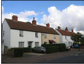
Figure 27 Rendered houses on northern section of Tennyson Road
