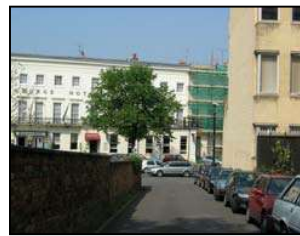
Figure 12 Bayshill Villas Lane
