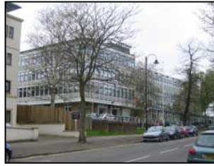
Figure 31 Rivershill House (Government Offices)
