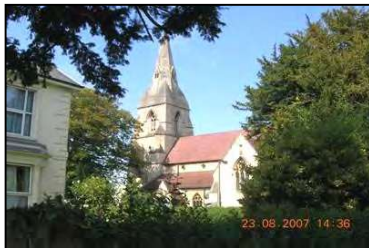
Figure 25 View of St Luke's Church from College Road
