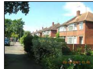
Figure 5 Semi-detached houses along the north side of Naunton Park Road
