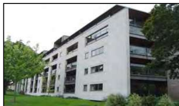
Figure 41 Century Court residential development on Bath Road
