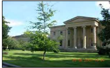
Figure 22 View of Thirlestaine House from Bath Road
