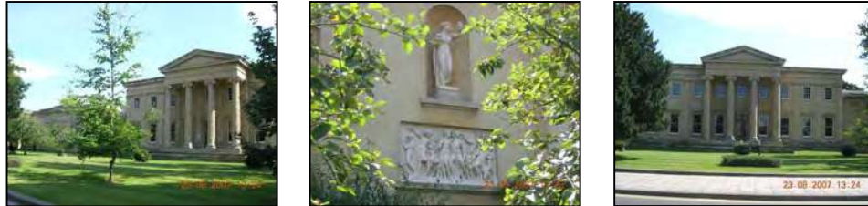
Figure 40 Detailing on Grade I listed Thirlestaine House
