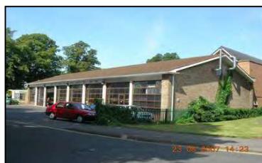
Figure 32 Cheltenham Fire Station
