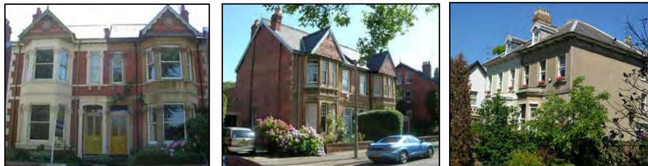
Figure 19 Unifying architectural detailing on houses
