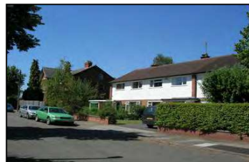
Figure 21 20 th century infill development
