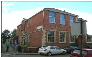
Figure 26 – St Paul's Church Centre, Swindon Road
