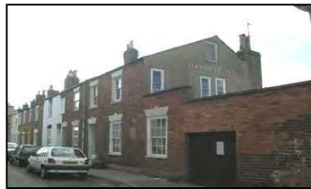
Figure 9 – High red brick wall on Hanover Street
