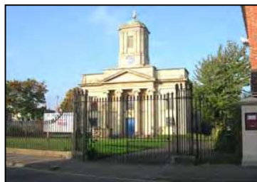
Figure 43 – Greenery around St Paul's Church
