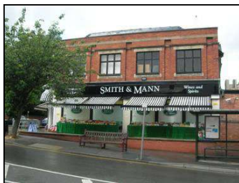
Figure 43 Smith & Mann traditional shop front, 41 a & b Lyefield Road West
