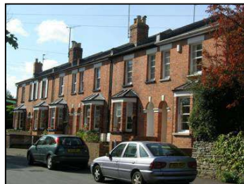
Figure 38 Red-brick terraced houses on Horsefair Street
