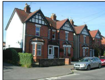
Figure 37 Distinctive semi-detached houses on Lyefield Road East
