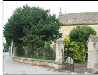
Figure 22 Listed railings and gate piers around St Mary's Church
