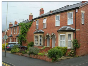
Figure 36 Unifying features on houses along Copt Elm Road
