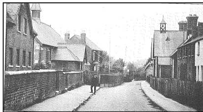
Figure 13 School buildings on School Road, no date
