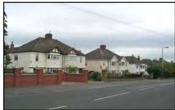
Figure 12 Semi-detached houses along Hatherley Road
