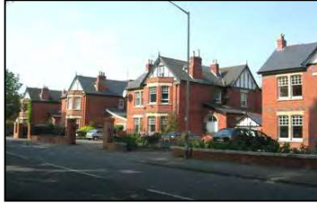
Figure 15 Hard-standing outside Edwardian houses on Hatherley Road
