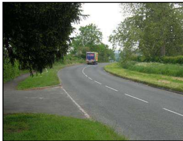
Figure 3 Southam Road forms part of the B4632
