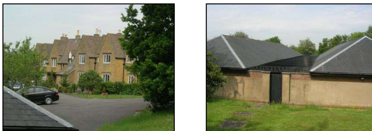
Figure 23 Residential development in the grounds of The Hayes and unattractive car port within the grounds
