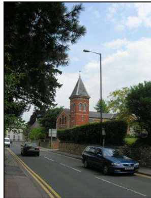
Figure 19 View along Deep Street with the United Reformed Church to the right
