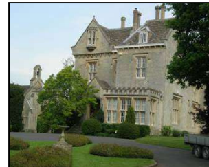
Figure 26 Architectural detailing on The Hayes
