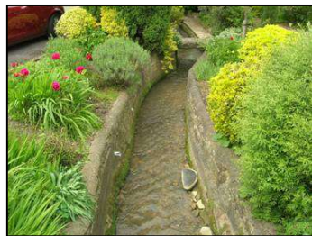
Figure 38 Stream forms part of the northern boundary of the Conservation Area
