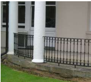
The colonnade at the rear of Hygeia House provides the earliest accurately dateable ironwork in the town
