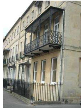
Examples of varying designs of ironwork between area railings, handrails and balconies/verandahs
