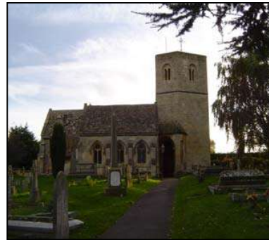
Figure 15 Church of St Lawrence
