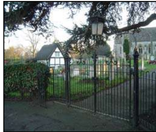
Figure 30 Pedestrian gates at Churchyard
