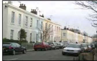
Figure 14 Front garden space along Prince's Road
