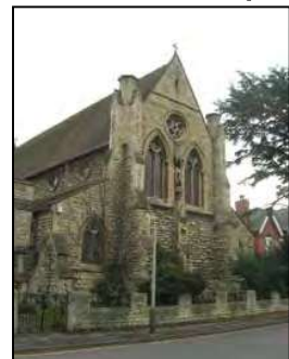
Figure 28 Detailing on St Stephen's Church
