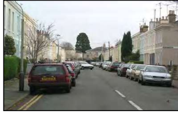
Figure 4 Example of terraced street – Prince's Road
