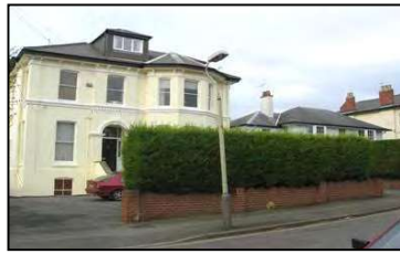
Figure 12 Villa on St Stephen's Road, with frontage converted into hard-standing
