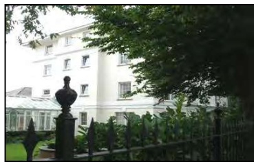
Figure 48 Greenery within Pegasus Court residential development
