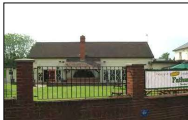
Figure 36 – The Norwood public house garden
