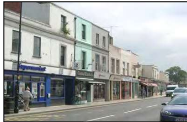
Figure 3 Shops along Bath Road with residential accommodation above
