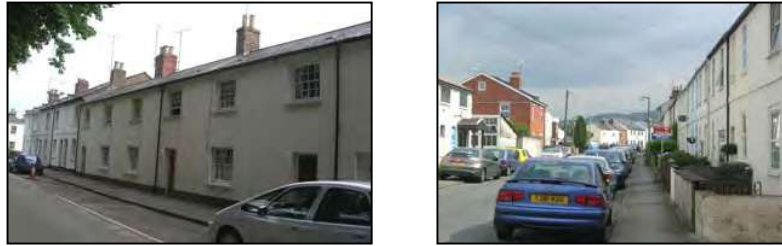
Figure 23 Historic terraced houses within Bath Road Character Area
