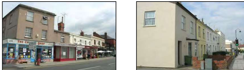
Figure 24 Mix of historic terraced buildings along Bath Road
