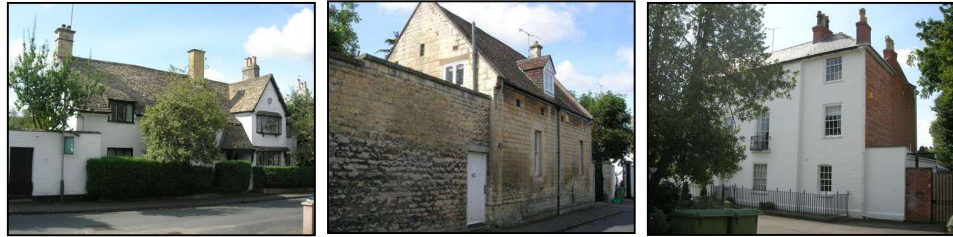
Figure 32 Architectural detailing on historic buildings in Cudnall Street Conservation Area
