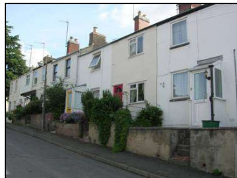
Figure 4 Residential houses on Hamilton Street
