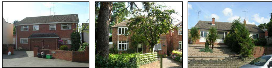
Figure 35 Modern developments on Cudnall Street Conservation Area
