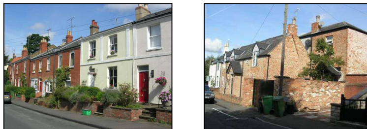
Figure 33 Red brick and rendered cottages along Cudnall Street
