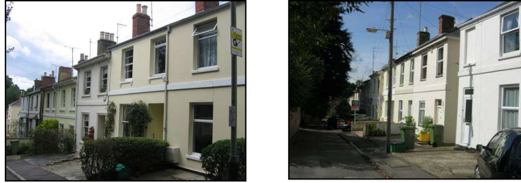
Figure 34 Terraced houses on Brookway Road
