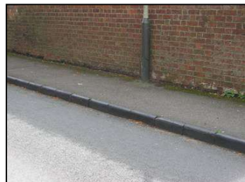
Figure 38 Historic kerb stones line Cudnall Street
