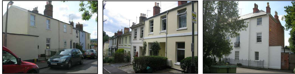
Figure 27 Residential properties in Cudnall Street Conservation Area
