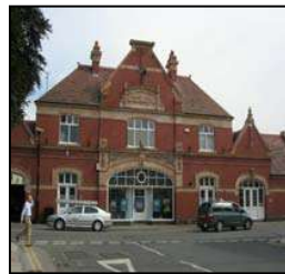
Figure 28 The Crescent Bakery building
