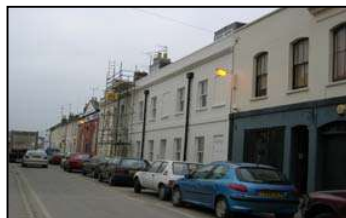
Figure 22 Terraces in Bennington Street
