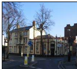
Figure 31 St James Hotel building
