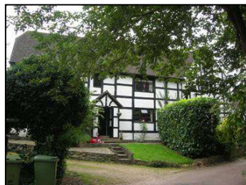
Figure 25 Timber framed Bafford Farm
