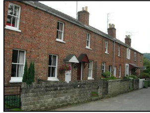
Figure 15 Low walls enclose the red-brick terrace on Bafford Lane
