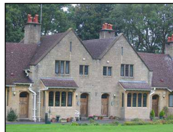
Figure 26 Stone mullion windows present on Bucklehaven almshouses
