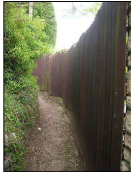
Figure 34 One of the footpaths in the Conservation Area
