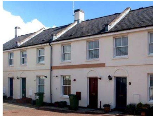
Fig.24 Modern terrace with roof articulated by party fire walls, Royal Oak Mews
