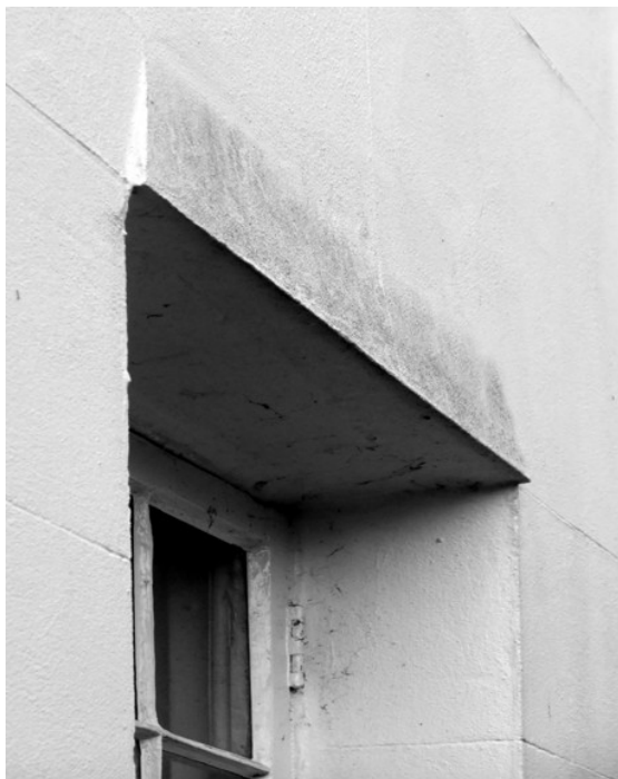
Fig.12 A bellcast moulding, Suffolk Parade
