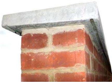
Fig.22 Once weathered coping, Queens Lane
