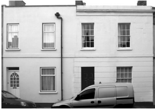
Fig.14 The effect on appearance due to the loss of original entablature, windows and door, St Paul's Street North
