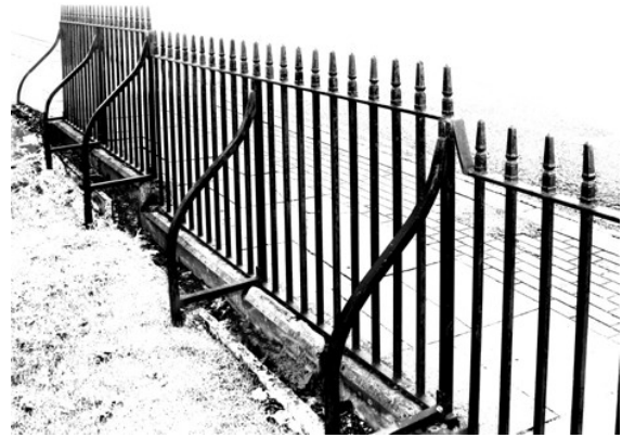
Fig.17 Railings inappropriately stepped, Montpellier Avenue
