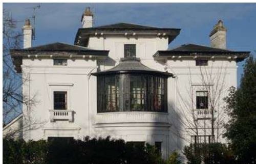
Fig.15 Projecting, bracketed eaves, The Park
