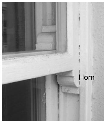
Fig.10 Victorian sash detail, Suffolk Parade
