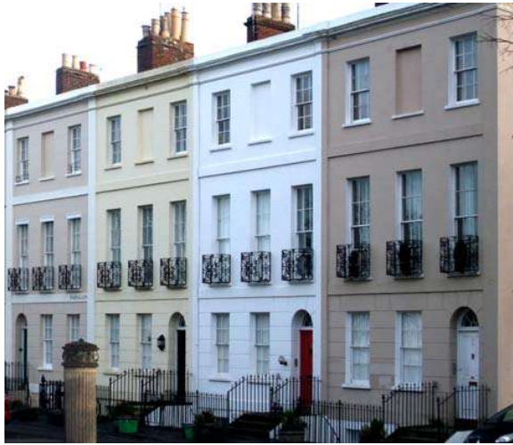
Fig.28 Painting each house differently in a small, informal street can appear attractively cheerful, but it detracts from a formal terrace such as this, especially where the pilasters are split between two colours, Bath Road
