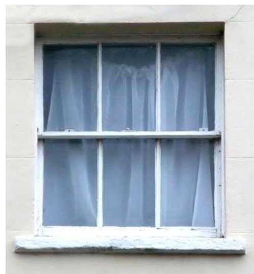
Fig.2 Square window with three panes per sash, Montpellier Retreat
