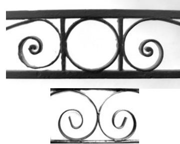
Fig.20 Regency wrought ironwork (top) and 20 th Century bent mild steel (below), Suffolk Parade
