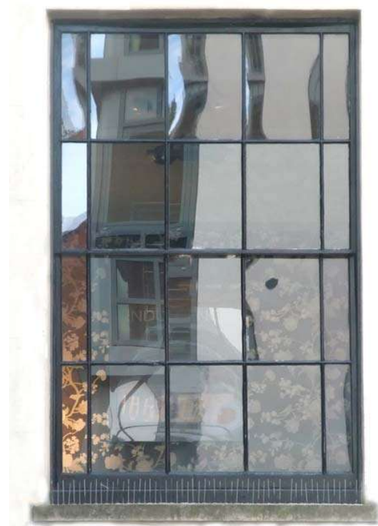
Fig.7 Window with marginal panes, some original crown glass and possibly original paint tones, Imperial Lane.
