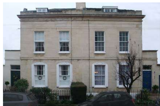
Fig.6 Doors to the sides of semi-detached houses allow windows to line through, but at the risk of duality, Montpellier Villas
