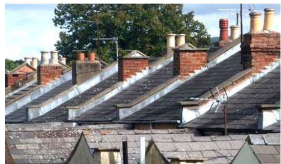
Fig.29 A nineteenth-century roofscape with external party firewalls, Swindon Street
