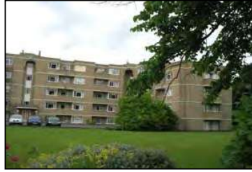
Figure 27 Suffolk House flats
