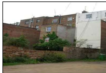
Figure 24 Rear elevations of terraced houses are frequently of exposed brickwork
