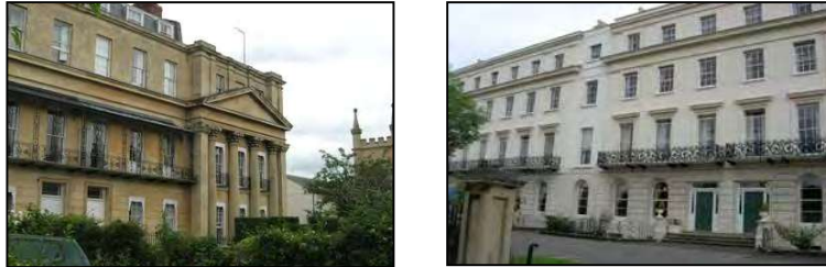
Figure 25 Balconies with Carron Company double-heart-and-anthemion motifs on Nos. 1-12 Suffolk Square (left) and Faithfull House (right)
