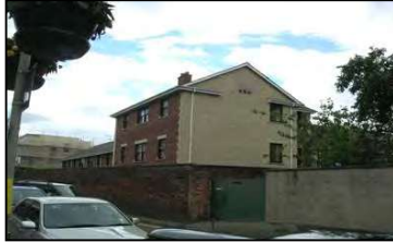
Figure 28 Suffolk Mews residential development
