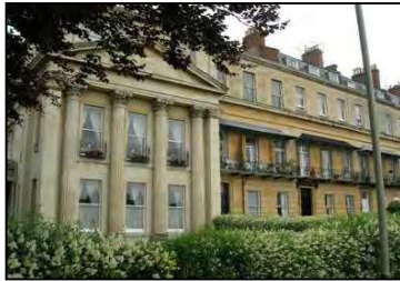
Figure 16 Historic terraced houses
