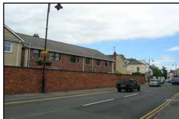
Figure 17 Suffolk Mews residential development
