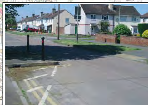
3. Uncontrolled pedestrian crossing point at traffic calming feature on Cromwell Road has dropped kerbs and tactile paving. Pedestrians only have to cross one lane of traffic.
