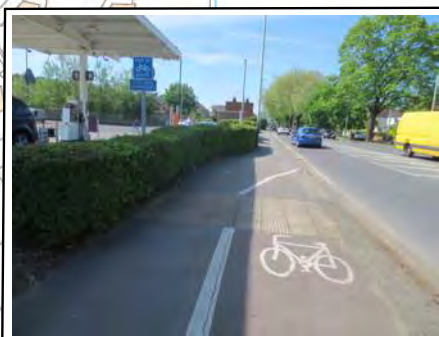
8. Existing shared footway / cycleway ends south of the signalised Priors Road / Redmarley Road junction. Cyclists are required to rejoin the carriageway.
