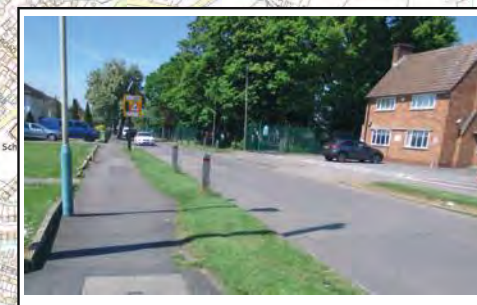
4. Lack of dropped kerb crossing points on Cotswold Road.
