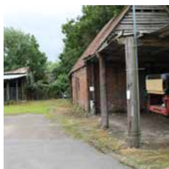
Fig.5.8 Barns at Swindon Manor Farm
