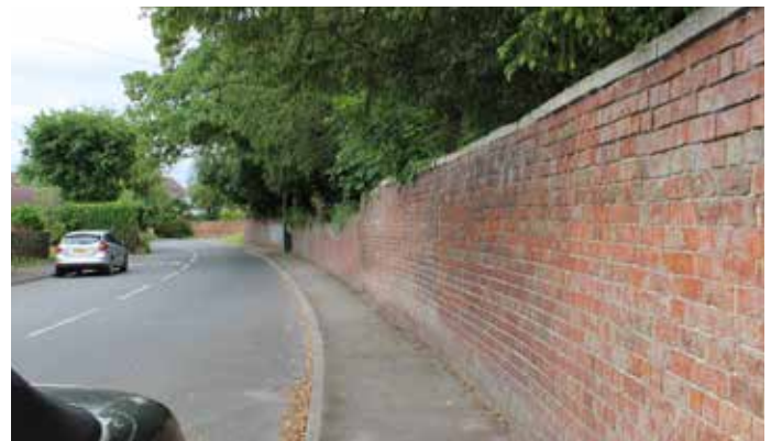
Fig.4.1. Historic Locally Listed boundary wall, Church Road
