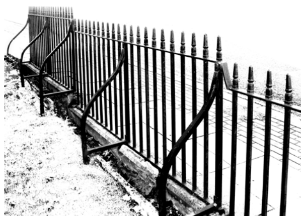
Fig.17 Railings inappropriately stepped, Montpellier Avenue
