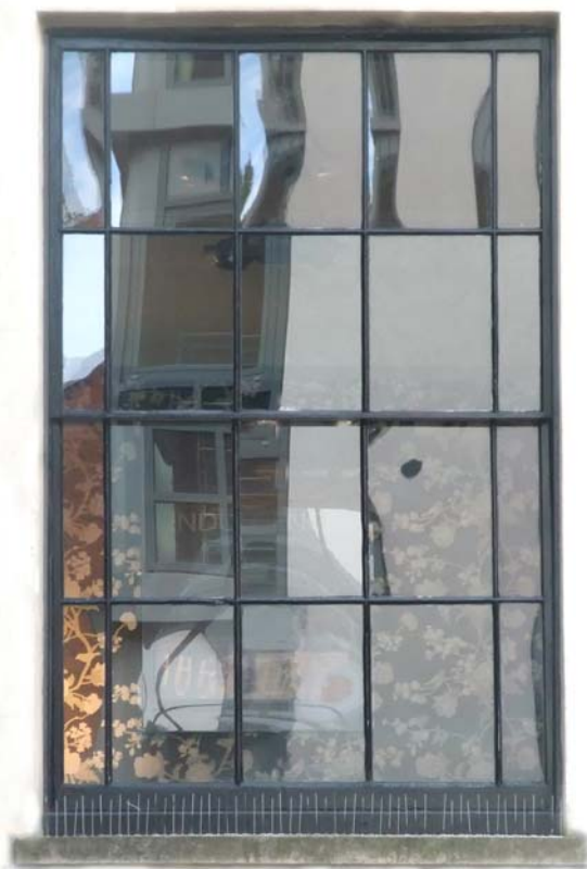
Fig.7 Window with marginal panes, some original crown glass and possibly original paint tones, Imperial Lane.
