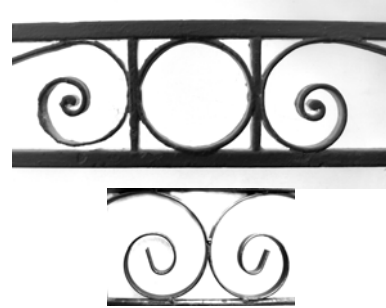
Fig.20 Regency wrought ironwork (top) and 20 th Century bent mild steel (below), Suffolk Parade
