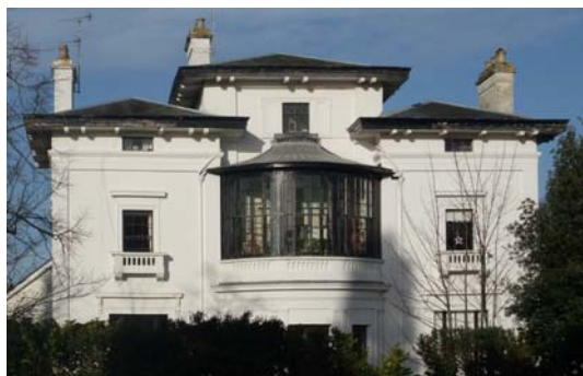
Fig.15 Projecting, bracketed eaves, The Park
