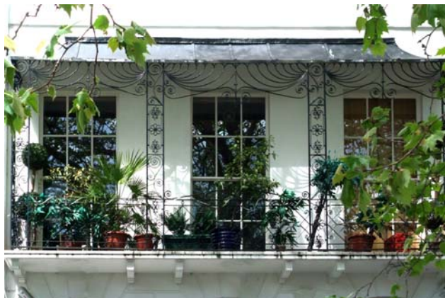
Fig.30 A well used, wrought iron Regency balcony, Cambray Place
