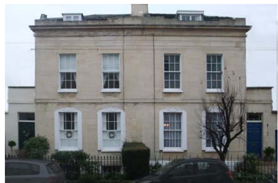
Fig.6 Doors to the sides of semi-detached houses allow windows to line through, but at the risk of duality, Montpellier Villas
