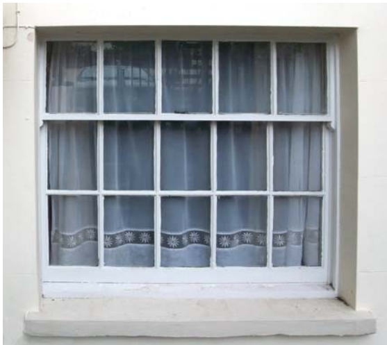
Fig.3 Unusually wide, horizontal window in a basement kitchen, Montpellier Retreat
