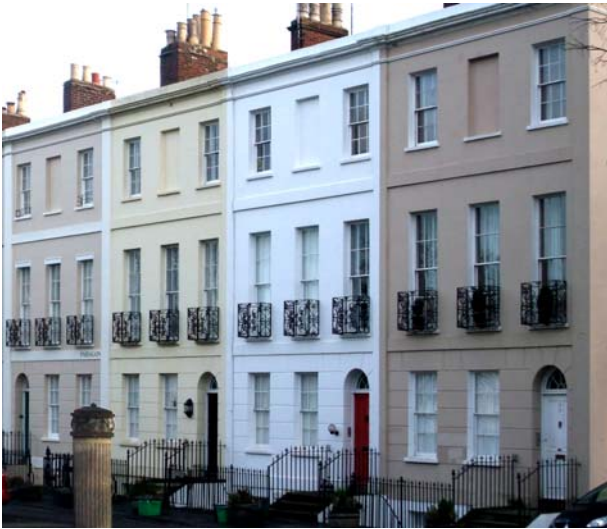
Fig.28 Painting each house differently in a small, informal street can appear attractively cheerful, but it detracts from a formal terrace such as this, especially where the pilasters are split between two colours, Bath Road
