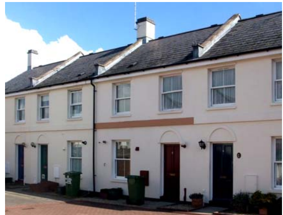
Fig.24 Modern terrace with roof articulated by party fire walls, Royal Oak Mews
