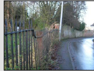
Figure 30 Part of the railings and wall along Mill Street
