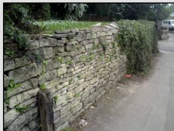
Figure 31 Part of Cotswold stone wall on east side of Deep Street
