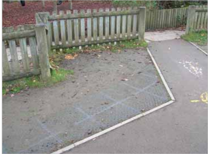
2007 worn grass in Evesham Road play area
