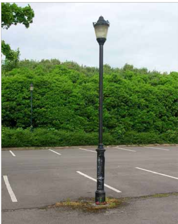
2007 Lighting in the Pump Room car park (above) and litter bin (below)
