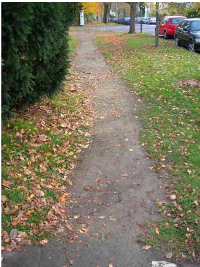
2007 Dirt track adjacent to Central Cross Drive
