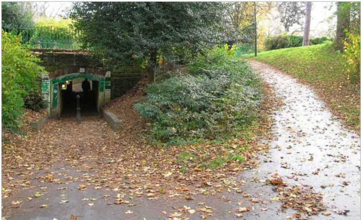
2007 Access into the park off Evesham Road.
